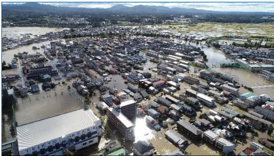
Flooded residential area (around Hidenoyama, Asakamachi)
