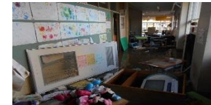
Three elementary schools damaged within city (Taken by Koriyama City)
