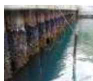
Deterioration of breakwaters
