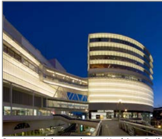
Commercial complex at Kashiwa Railway Station
