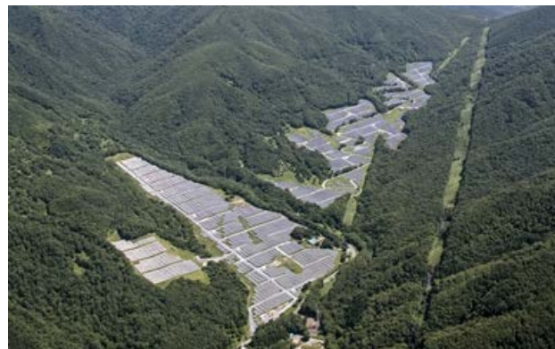
Goyozan Photovoltaic Power Generation Plant (generating capacity: 18MW)
