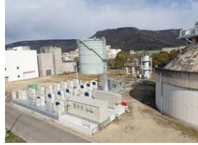
Biomass power generation facility
