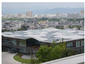
Gifu Media Cosmos that actively utilizes geothermal heat and solar light
