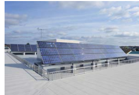
Solar panels installed at Kohan Elementary School: 10 kW
