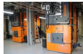
↑Wood biomass boilers
