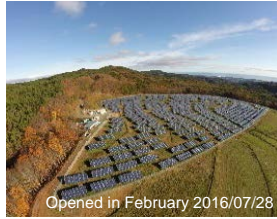
Opened in February 2016/07/28 Kaeu Kawauchi Mega Solar Power Plant
