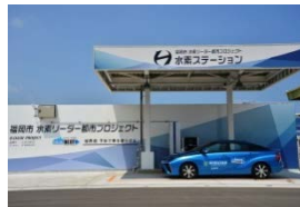
Sewage biogas hydrogen station
