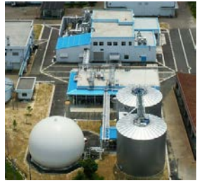
Garbage Biogas Generation Center
