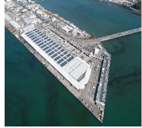
Solar power generation through roof rental in the Kochi City Wholesale Market
