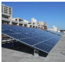
Solar power generation facility (installed on the roof of an elementary school)
