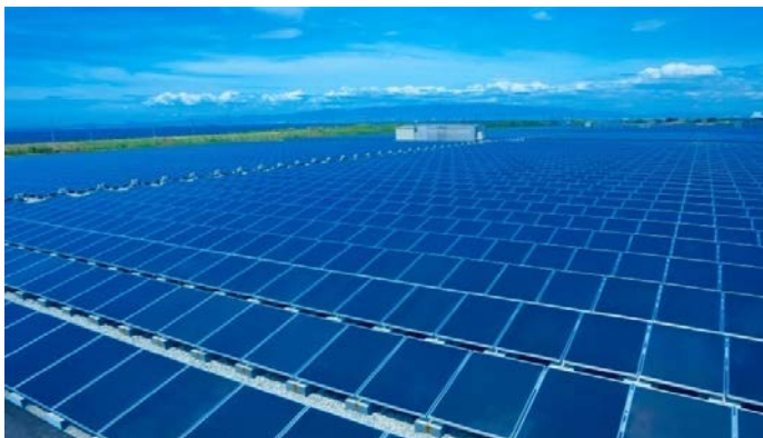
Sakai Photovoltaic Generation (10 MW)
