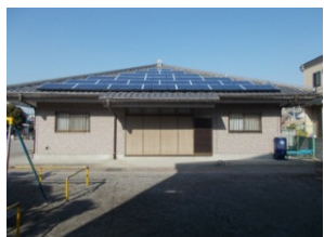
Photovoltaic generation system
