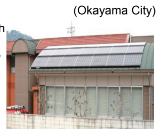
▲The 4th Civic Joint Power Plant ▲<Okayama Municipal Seto Town Library>
