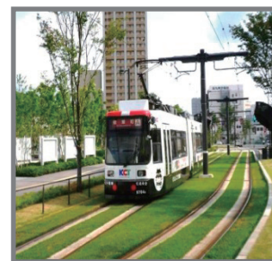
<▲Green carpet for street cars Greening of the street car track fields was implemented>
