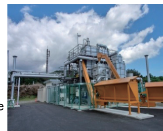
<Bio-methanol production and power generation facility>
