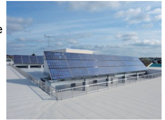
<Solar panels installed at Kohan Elementary School: 10 kW>
