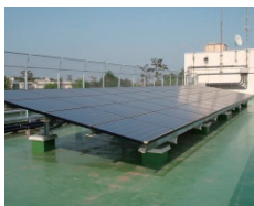
<The photovoltaic power system at a municipal school>
