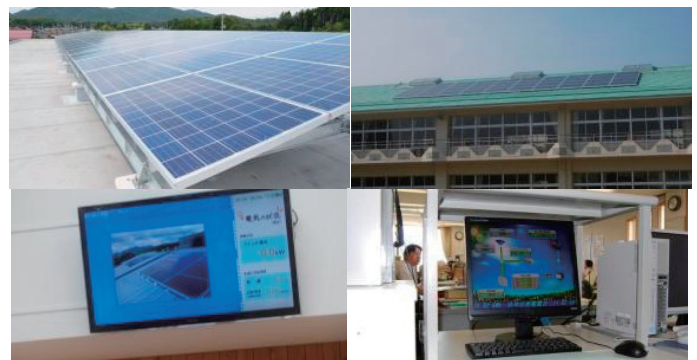
The photovoltaic generation systems installed in four elementary and junior high schools in town
