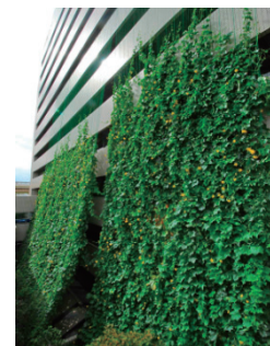
<Installation of green curtains in the public facility>
