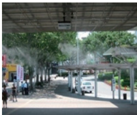
<Mist spray at South Exit of Kugagaya Station>
