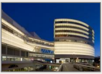
Commercial complex at Kashiwa Railway Station
