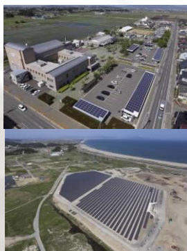
2014 Carport solar system established at the same time as mega solar through private investment
