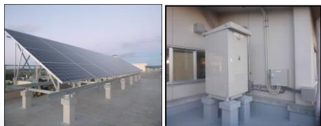
2011~2015 PV and storage batteries (GND) built in core shelters within the city
