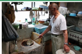
Geothermal hot-water supply
